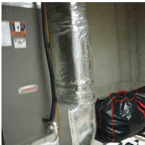
Mechanicals/unfinished basement area
