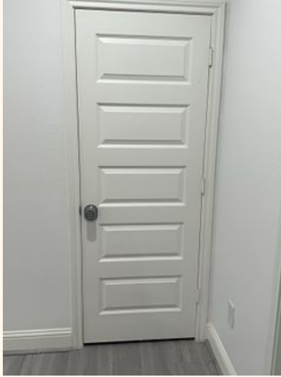
Second floor hallway
