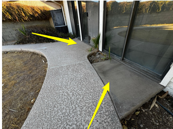
Example: surfaces slope toward structure
