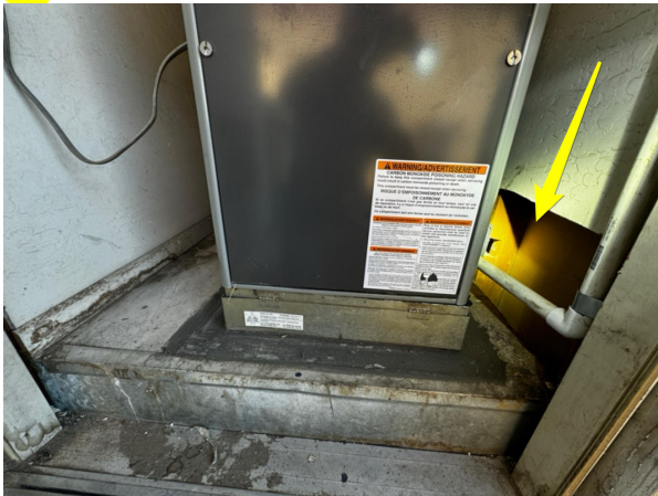
Example: wall cut open
