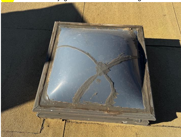
Damaged lens
