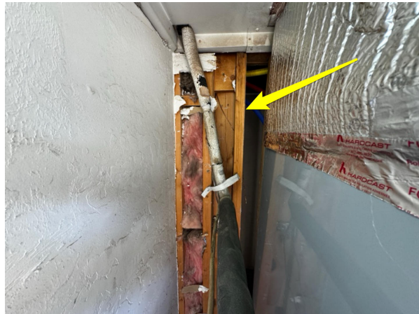
Example: wall cut open
