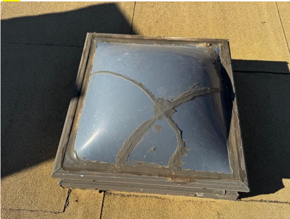
Damaged lens
