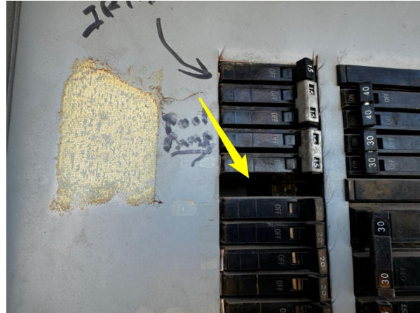
Knockout cap needed
