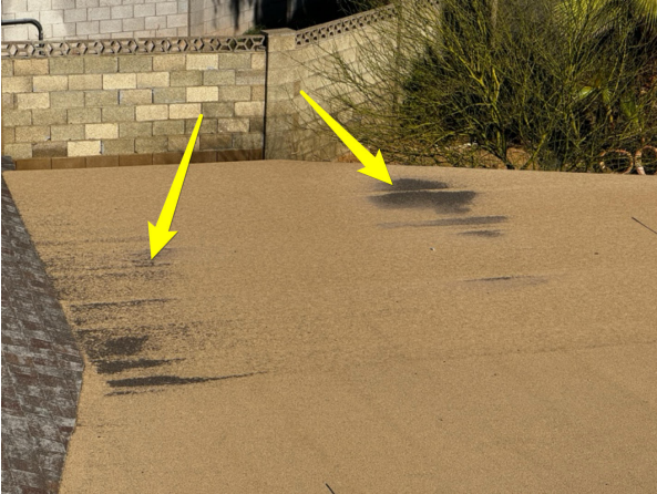
Example: granule accumulation
