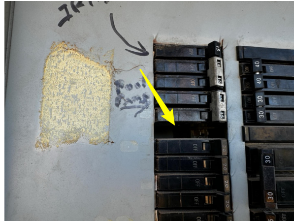
Knockout cap needed
