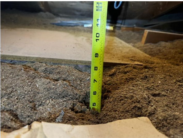
Example: low insulation
