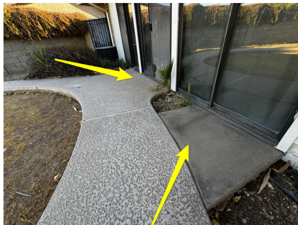
Example: surfaces slope toward structure
