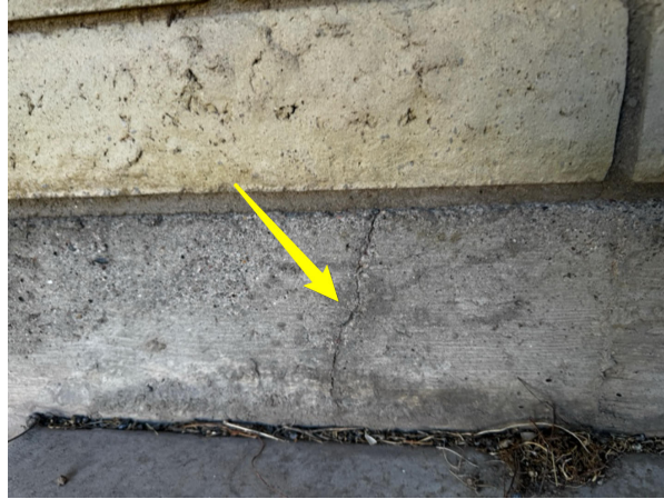
Example: crack
