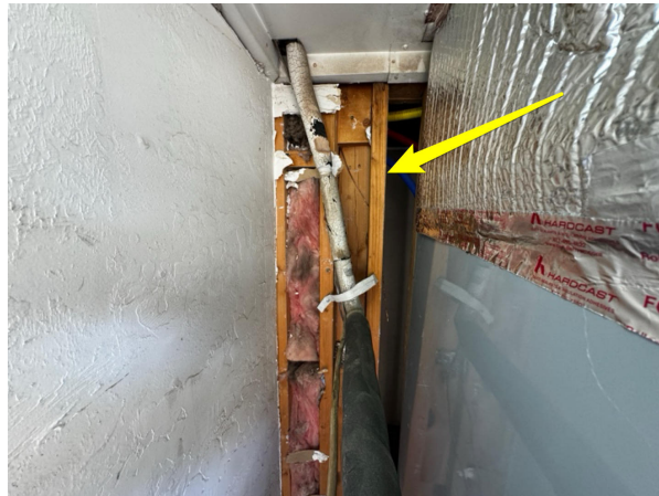
Example: wall cut open
