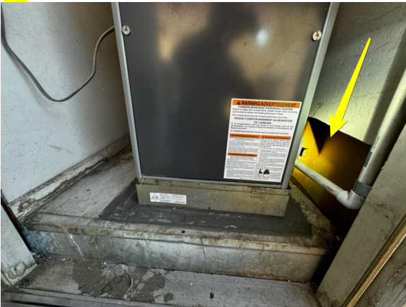
Example: wall cut open
