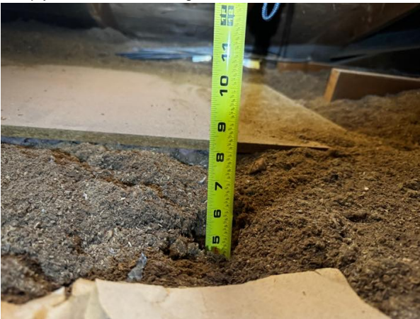
Example: low insulation
